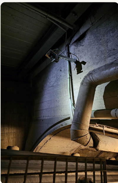
QUARRY • CROSS-SCAN OVER BELT
