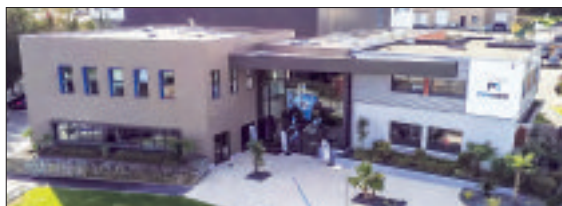
Front view of Palamatic Process after the 2023 extension.
