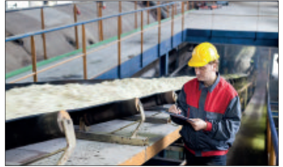
Powdered material travels along an inclined conveyor.
