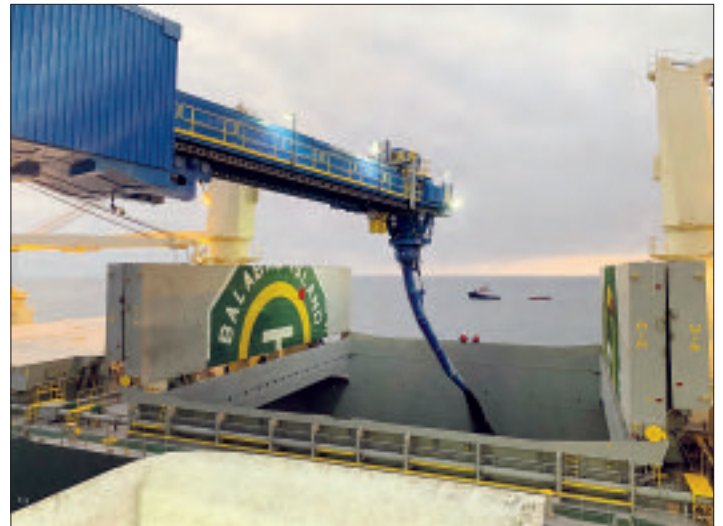
The material slides down a telescopic tube into the cargo hold.
