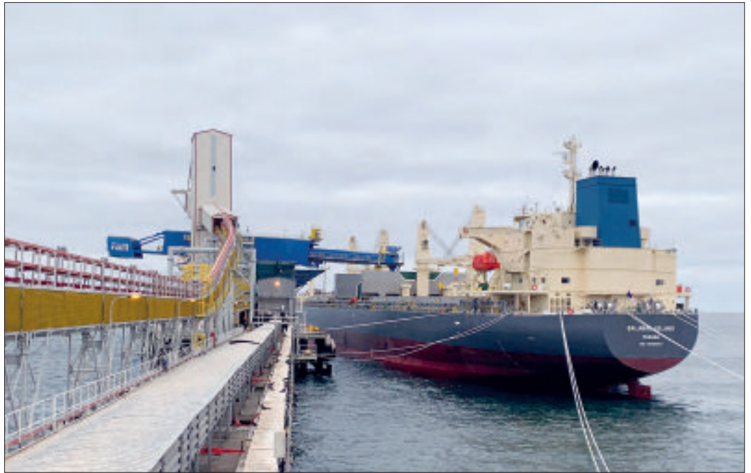
At the end of the boom is the loading device with a belt conveyor.
